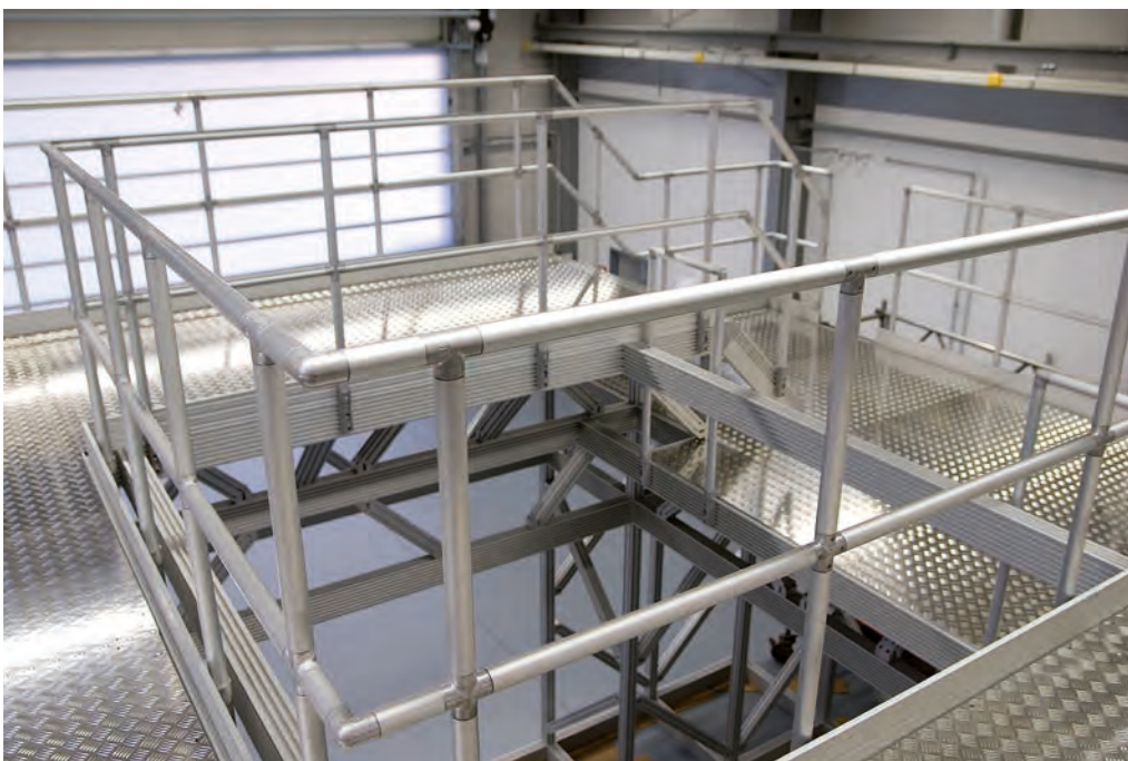
Working platform with ITAS railing
