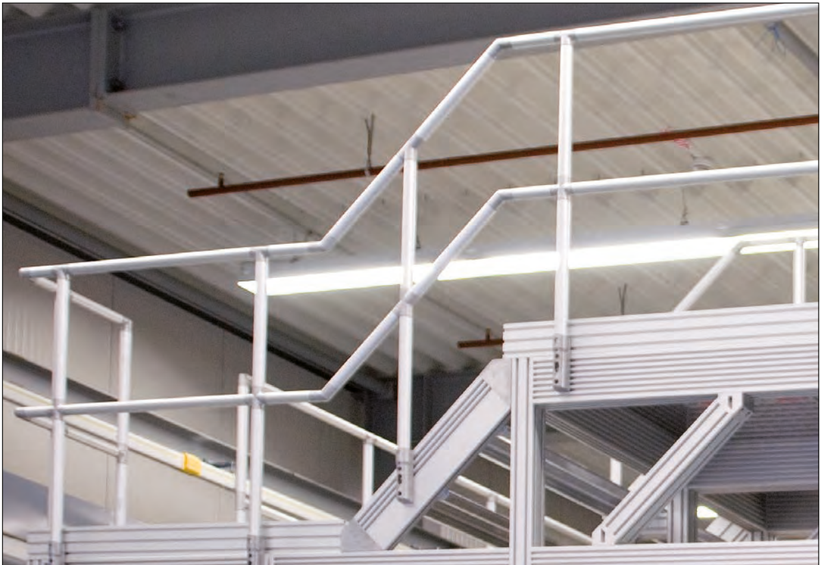
Staircase between two operating platforms.
