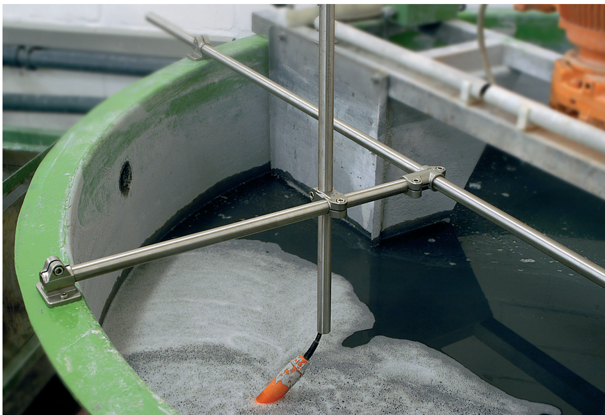
Simple probe fixation in an aggressive environment.
